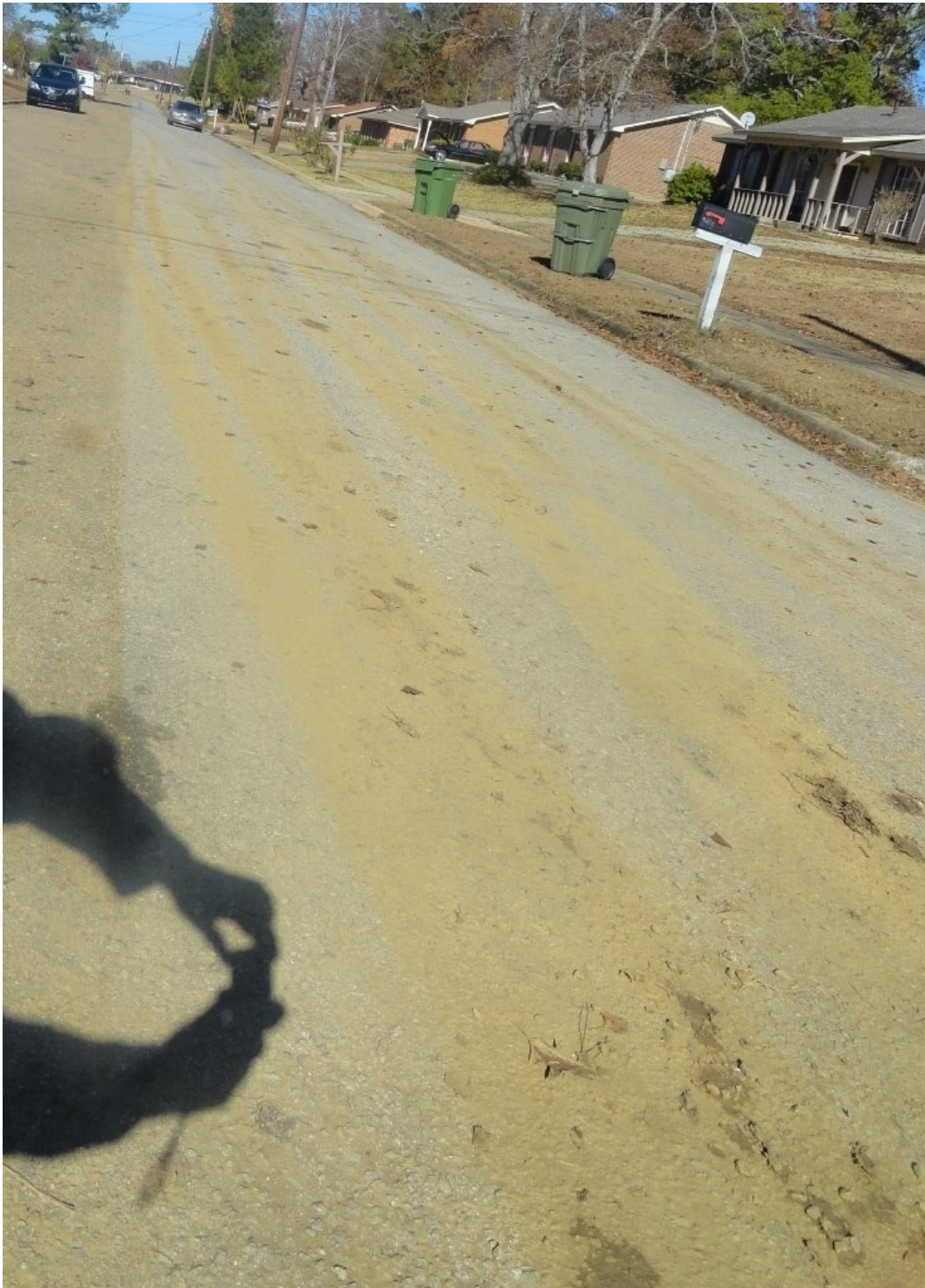
Sediment Tracking on Andova Drive 11.18.2013
