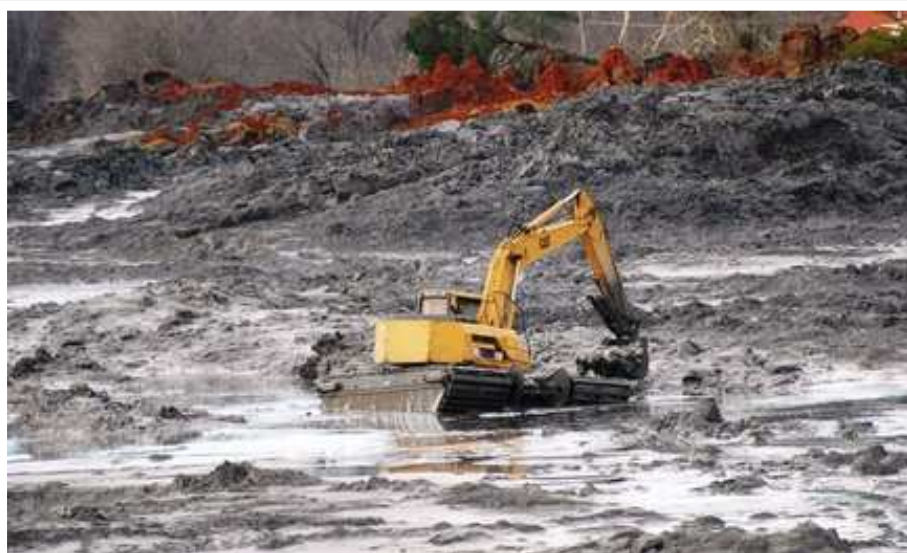
A trackhoe scoops up spilled coal ash which is being loaded into rail cars for shipment to an Alabama landfill in Perry County for disposal. (Special/TVA)
